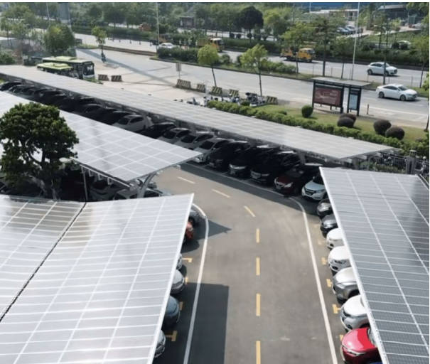
光儲充停車場 Parking Lot of PV System Coupled with Battery Storage and EV Charging Stations
