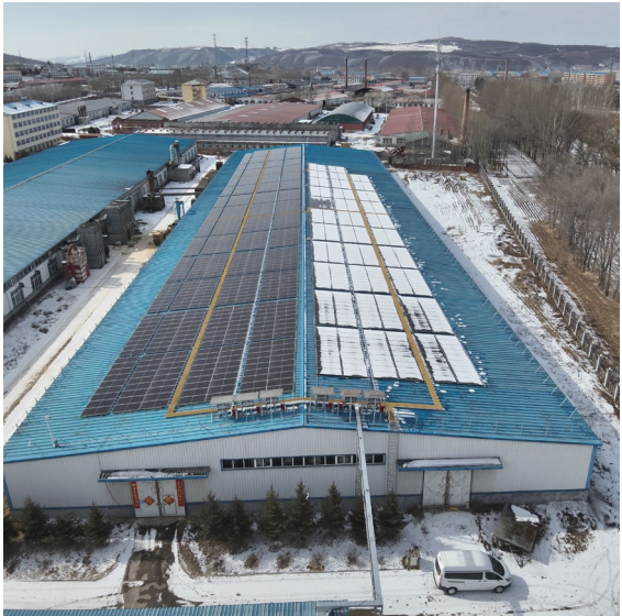
182 單晶單玻 545W 光伏元件 182 Single-crystal Lattice Single-layer 545W PV Component
